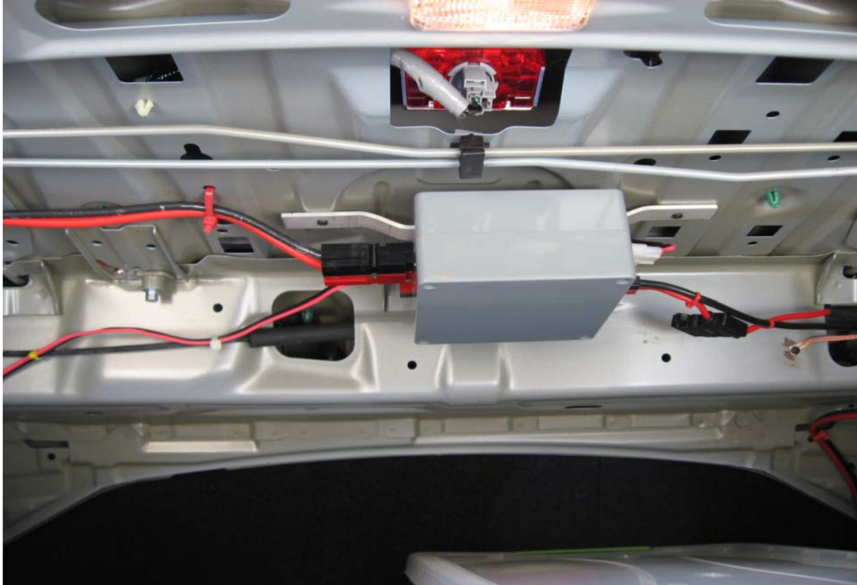
Figure 5. Trunk-mounted relay enclosure and cabling. The 8 AWG battery power feed enters the enclosure via the APP pair on the left. Behind it is the control input wiring from the panel switch shown in Figure 4. The 10 AWG power cable exiting to the right is protected by a 30A inline blade fuse. It's routed under the rear seat and carpet to the in-cab West Mountain 5x APP strip shown in Figure 6 on the next page. The enclosure and all cable ties are secured to the rear deck's metal understructure. Note the hard-point ground at the right – used to provide a solid ground for the antenna.
